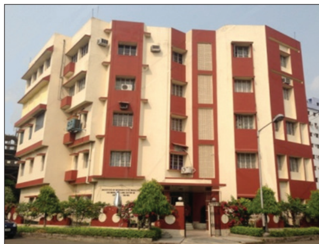
Fig-15: IRM new Building
