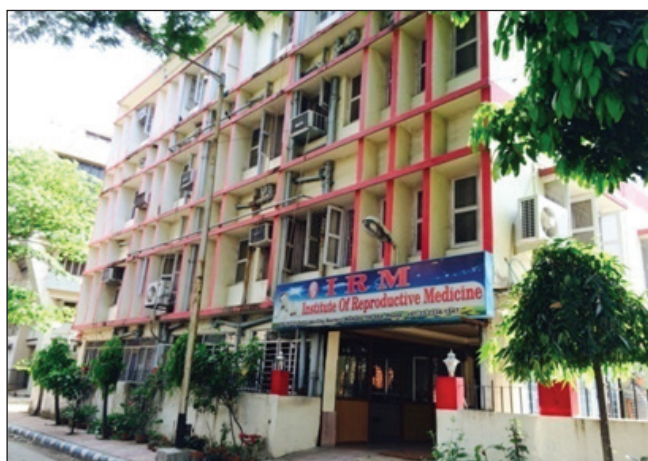
Fig-14: IRM Old Building
